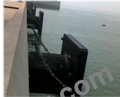
In the front it is equipped with a frontal frame which greatly reduce the face pressure on ship panel and the friction coefficient. Due to its structure, the product has the characteristic of higher force absorption and long usage life.
