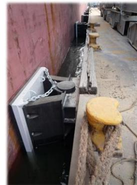
Unit Element Fenders are a high performance, modular system. Element Fenders can be combined in unlimited permutations of length, orientation and Energy Index to suit a wide variety of applications. The simplest Unit Element system is the UE-V fender which employs pair(s) of elements and a structural UHMW-PE face. UE-V fenders combine high energy capacity with low friction face and high wear resistance.
